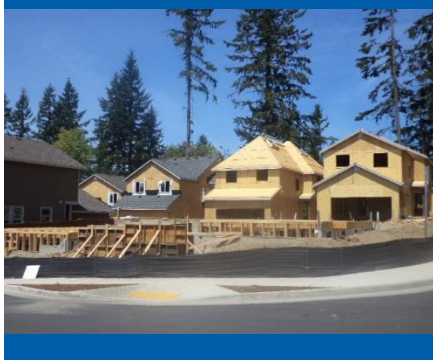
Construction of Summer Falls, one of Beaverton's newest subdivisions
